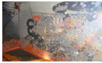
Mechanical power tool de-rusting ST2-3 followed by high pressure freshwater washing.
