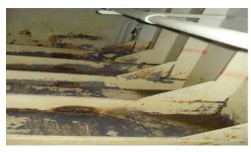
Mechanical power tool de-rusting before high pressure washing.
